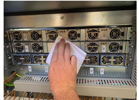
Figure 9-13 Wipe Around Fans
