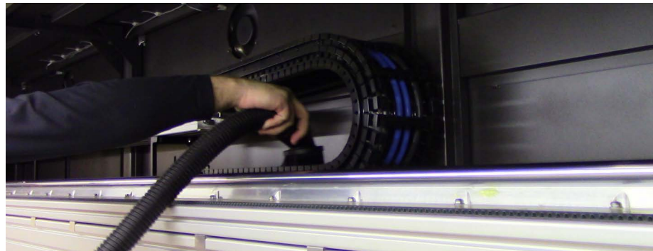
Figure 9-4 Vacuuming umbilical assembly
