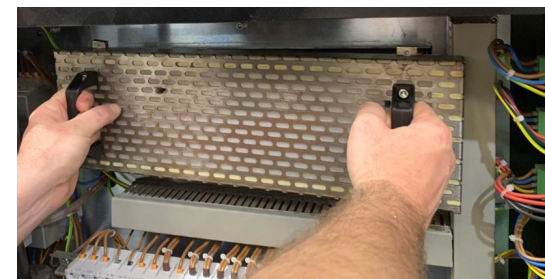
Figure 8-2 Power Supply Filter Assembly
