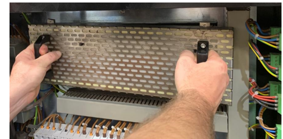
Figure 9-11 Power Supply Filter Assembly
