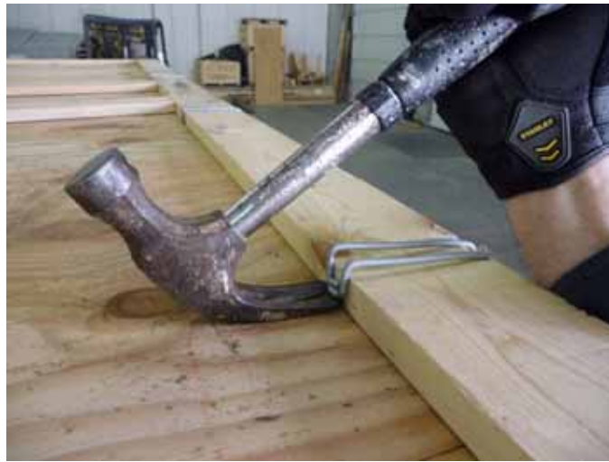
Figure 4-2: Retaining Clips
