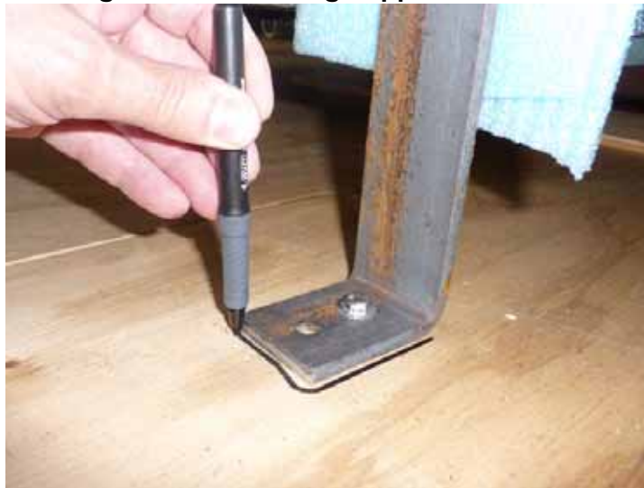
Figure 4-7: Marking support locations
