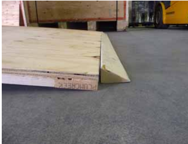
Figure 4-6: Wedge at ramp end
