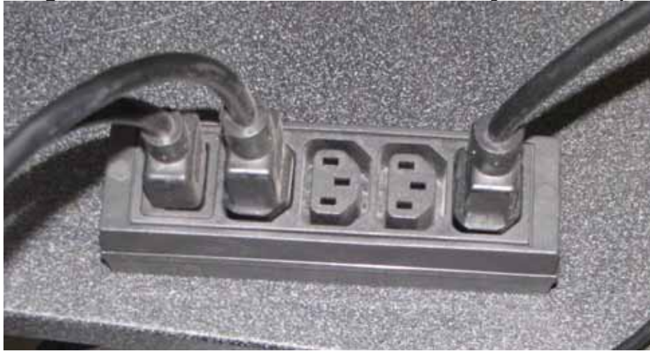
Figure 17: T1000 220VAC Dedicated Auxiliary Power Strip
